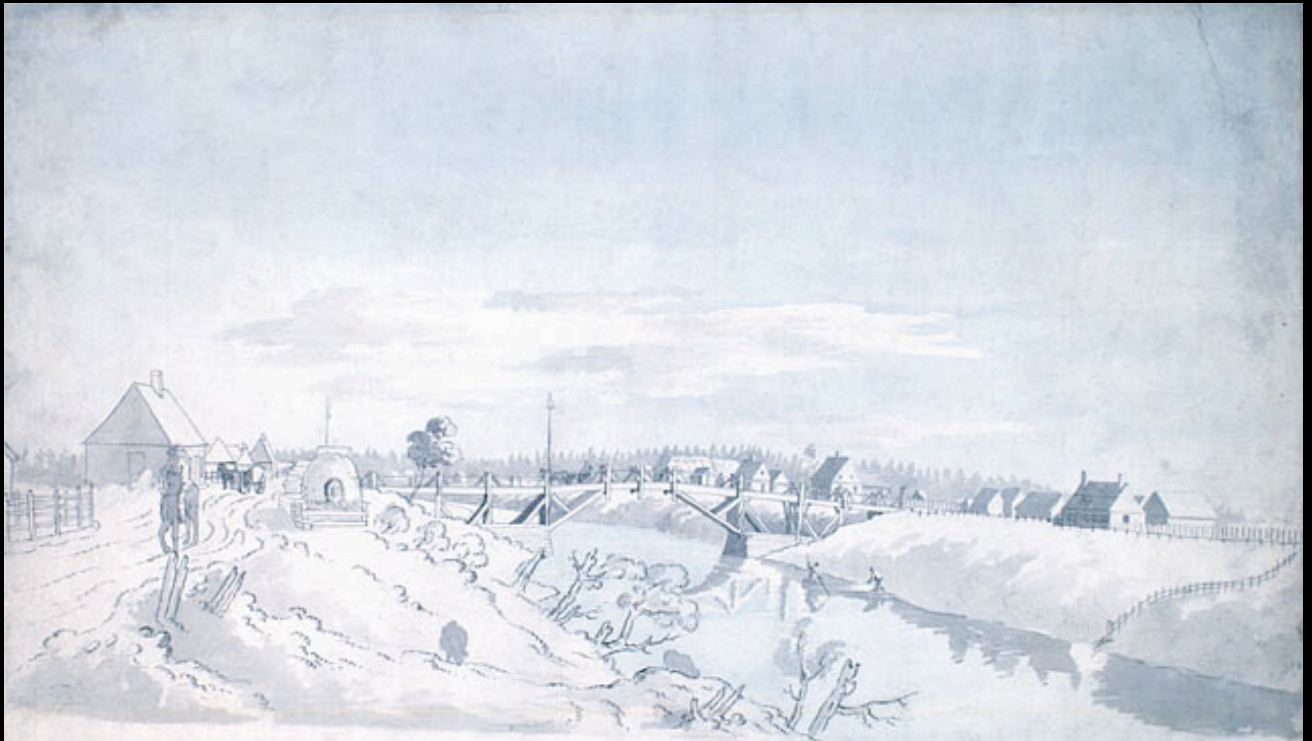
A View of the Bridge at Rivière de Loup taken from the South West
