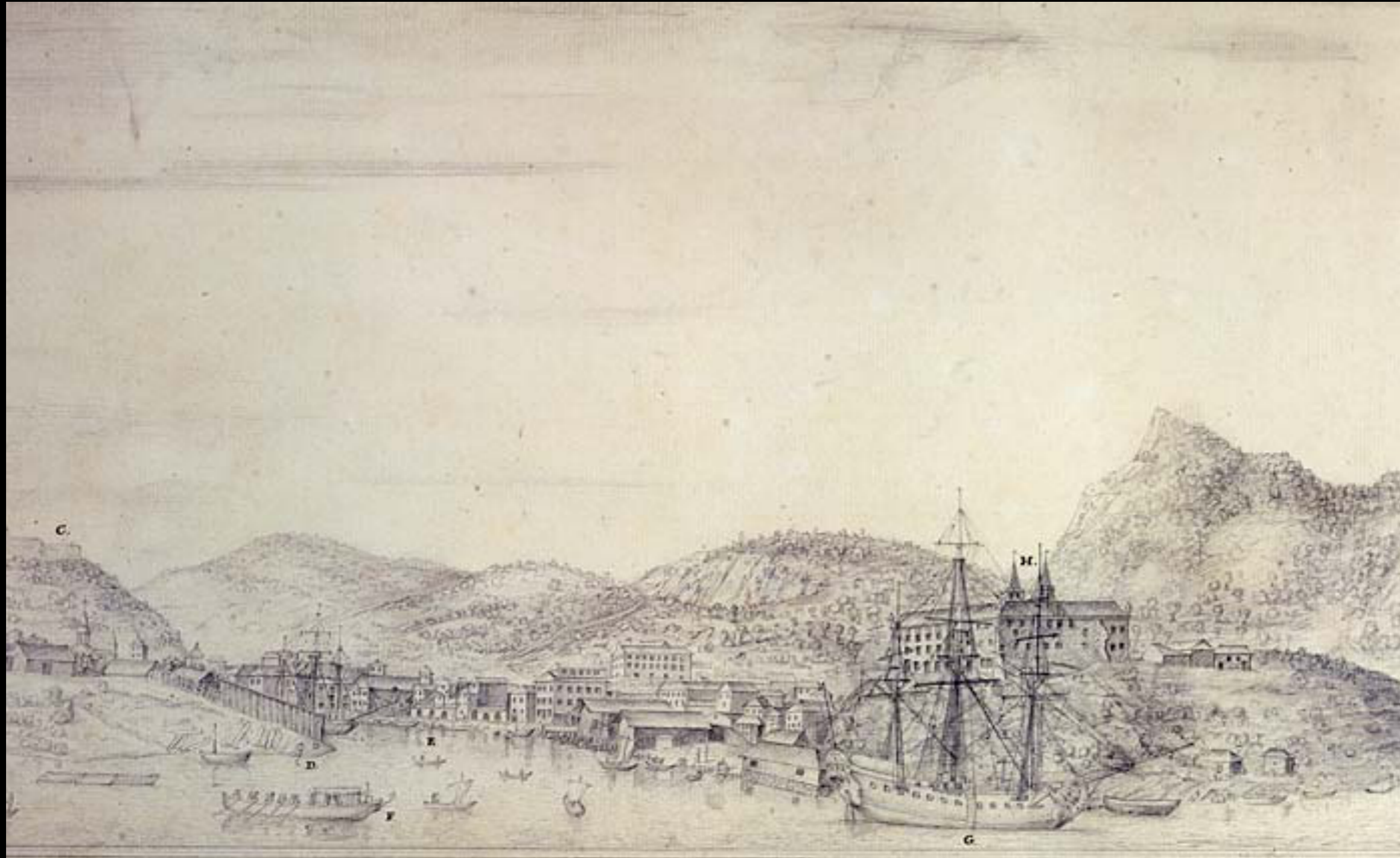
A VIEW of the Town of RIO JANEIRO from the Anchoring-Place.
