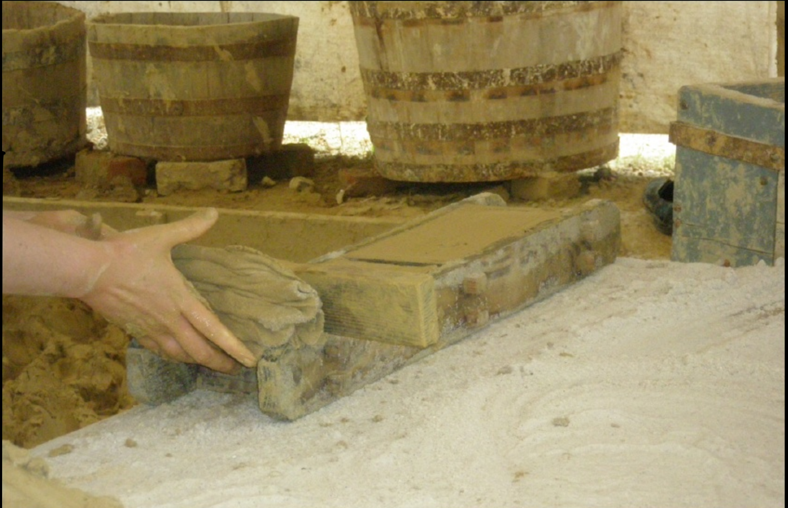
Recreated Brick Maker forming a Brick in a Wooden Mold (Colonial Williamsburg)
