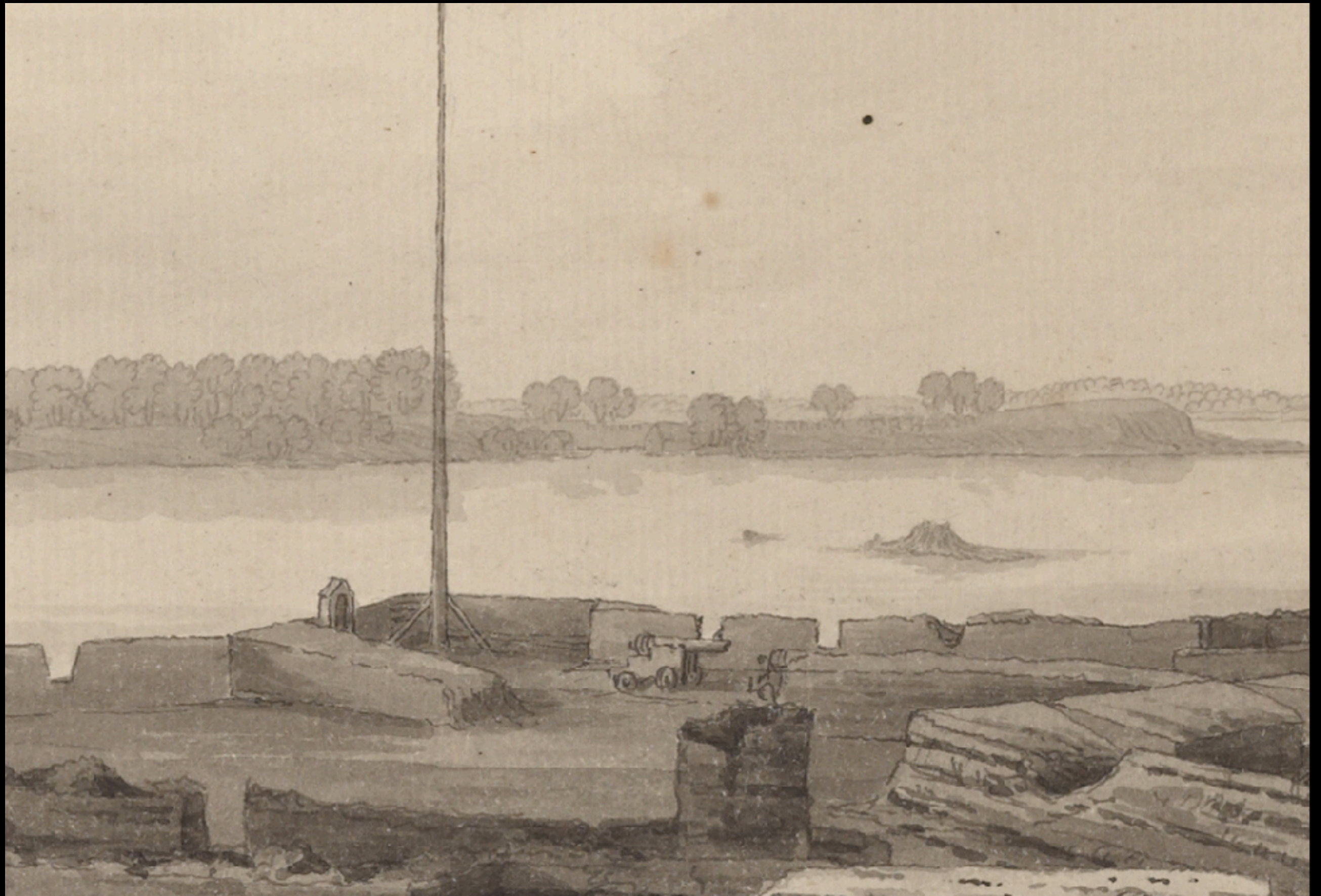
“View of the rebel work round Walton's House, with Hell Gate & the Island [illegible]” by Captain Archibald Robertson, British Engineers (New York Public Library)
