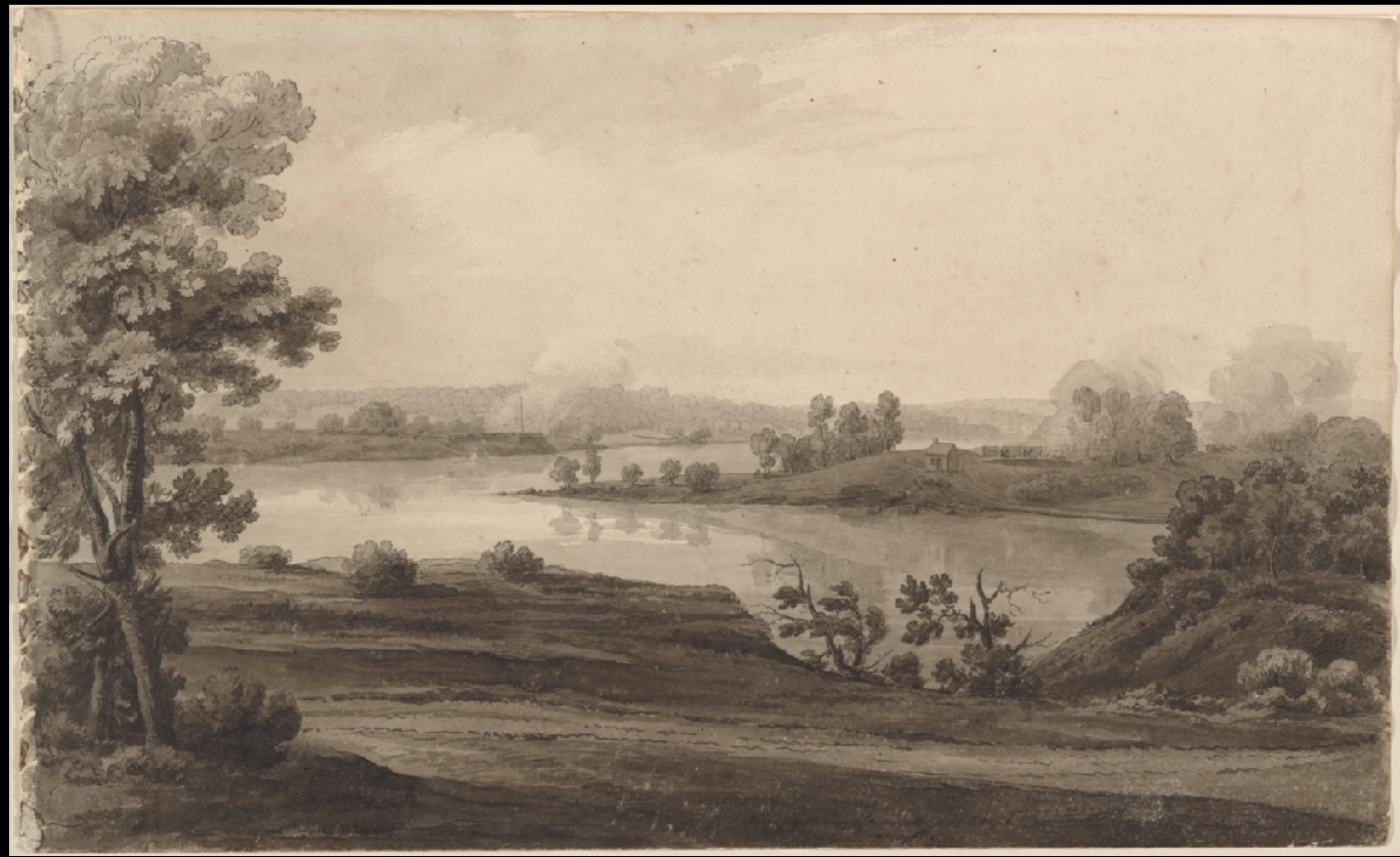
“View of the opening of our Batterys at Hell Gate upon the rebel works around Walton's House on the island of N. York. 8 Sept. 1776” by Captain Archibald Robertson, British Engineers 8 September, 1776 (New York Public Library)
