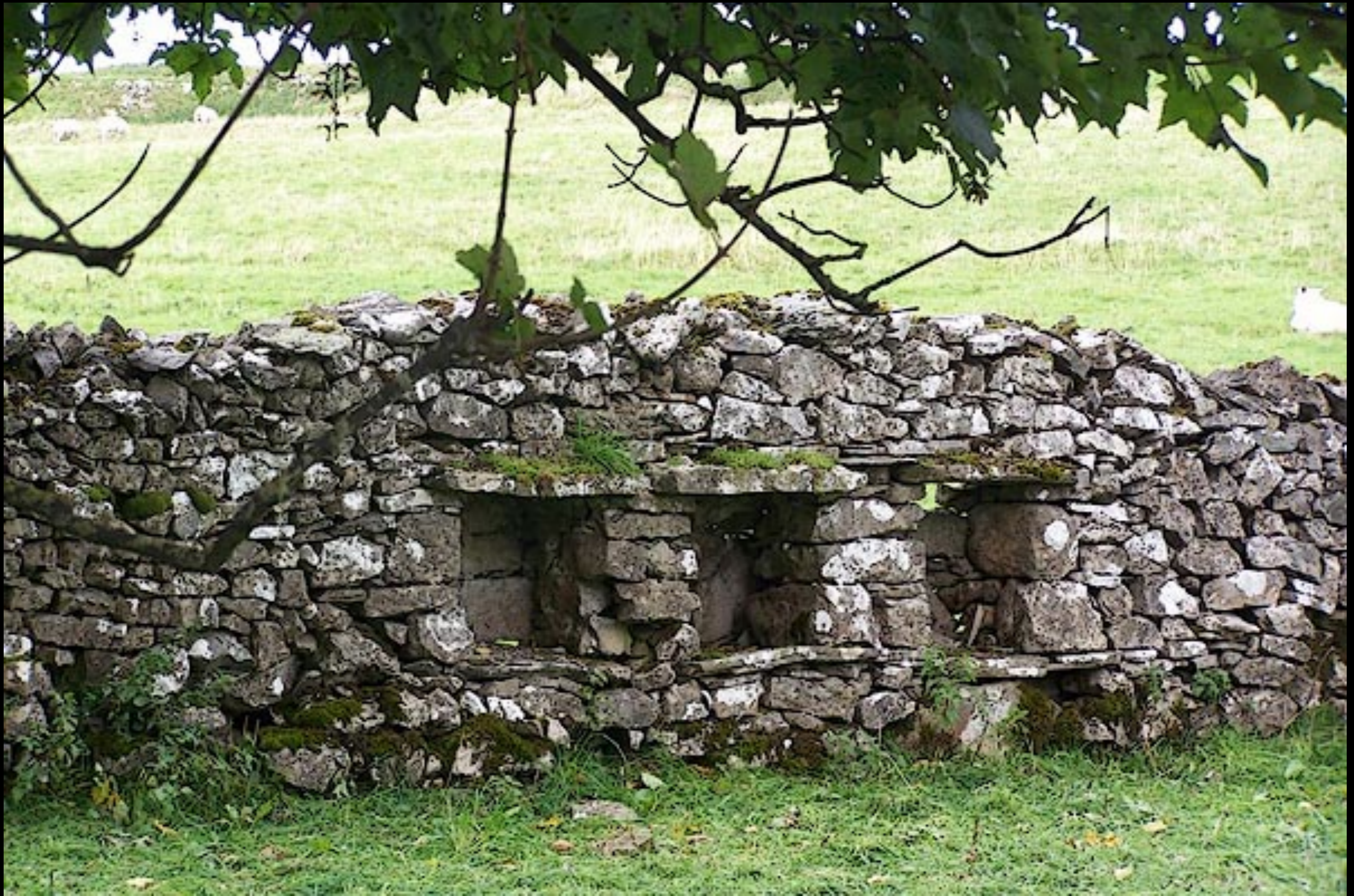
English "Bee Boles" Built into a Stone Wall to Keep Bee Skeps Out of the Rain Westmoreland and Cumberland - Late 17th to 18th Century (Public Domain)
