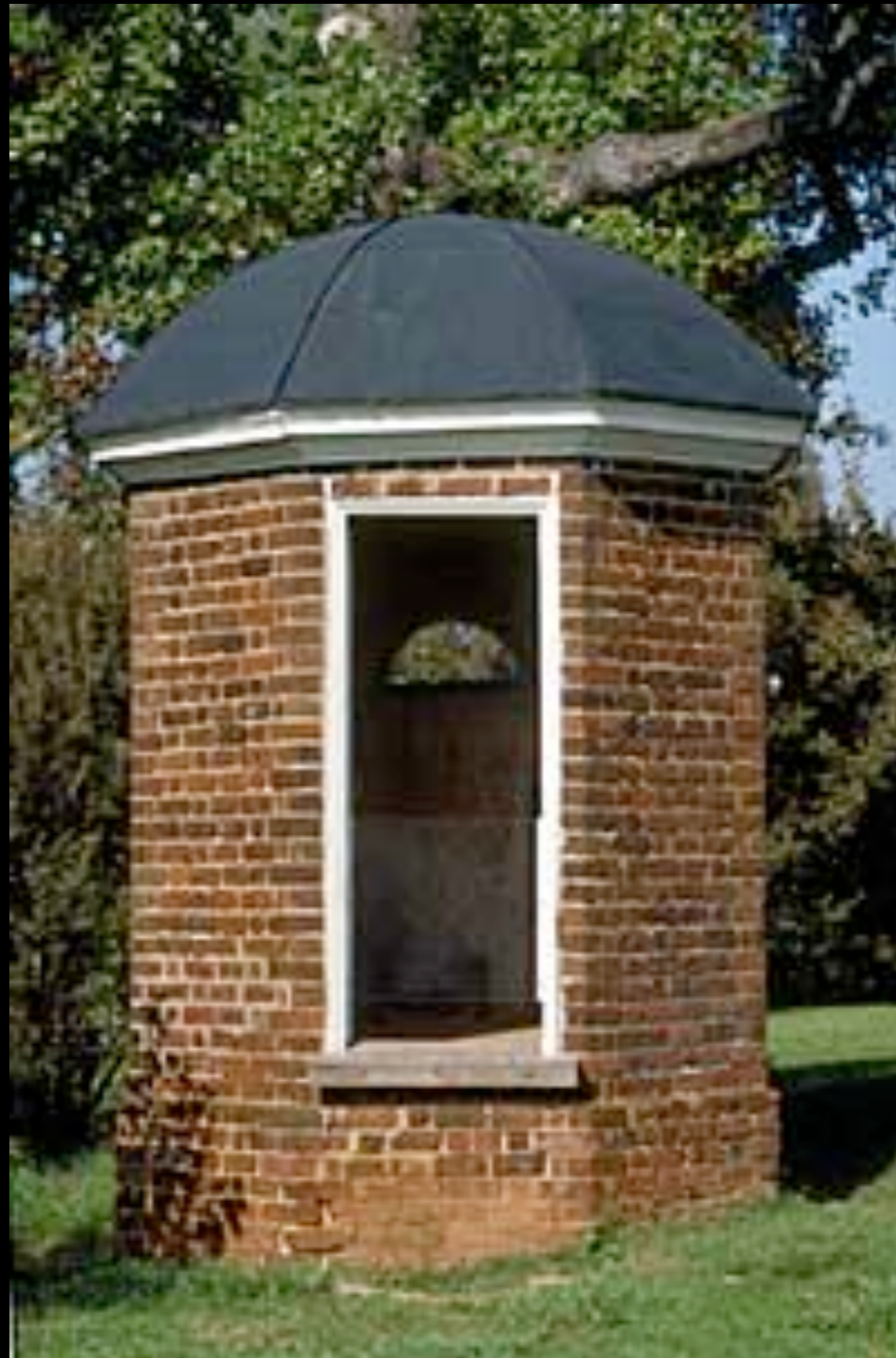
Brick Privy Built by Thomas Jefferson at His Retreat, Poplar Forest
