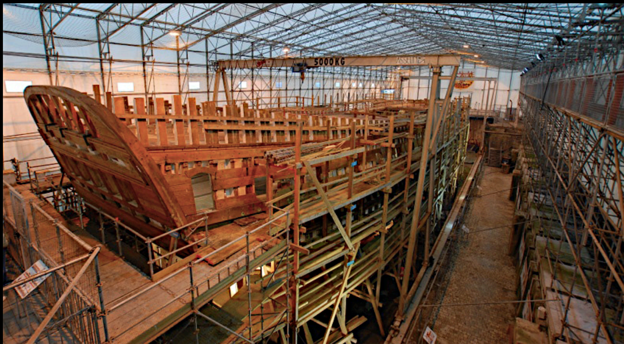
Reconstructing L'Hermione - Rochefort, France
