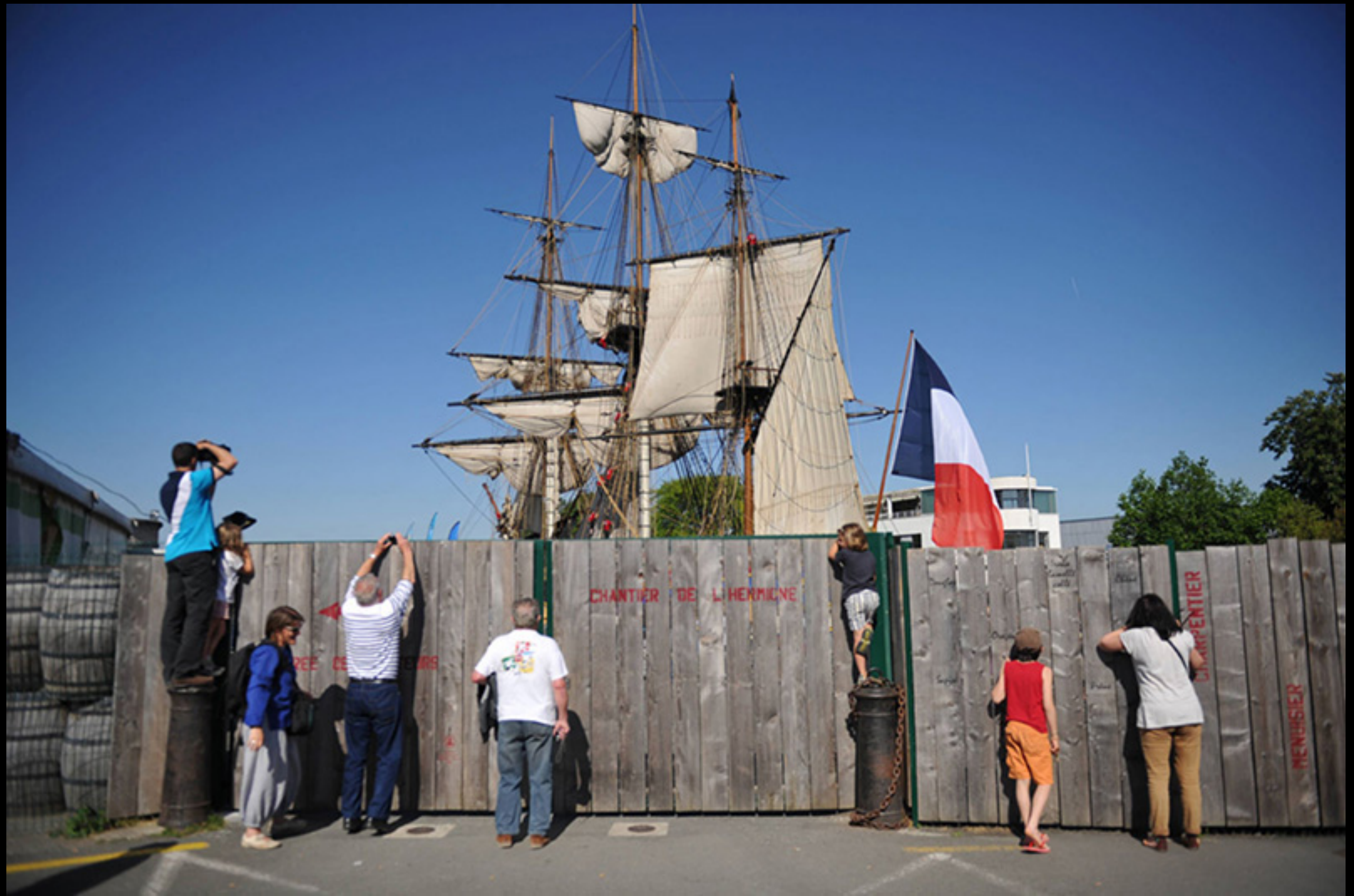
Reconstructing L'Hermione - Rochefort, France
