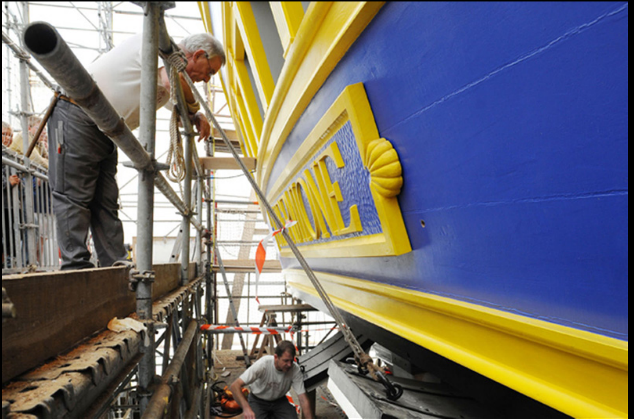
Reconstructing L'Hermione - Rochefort, France
