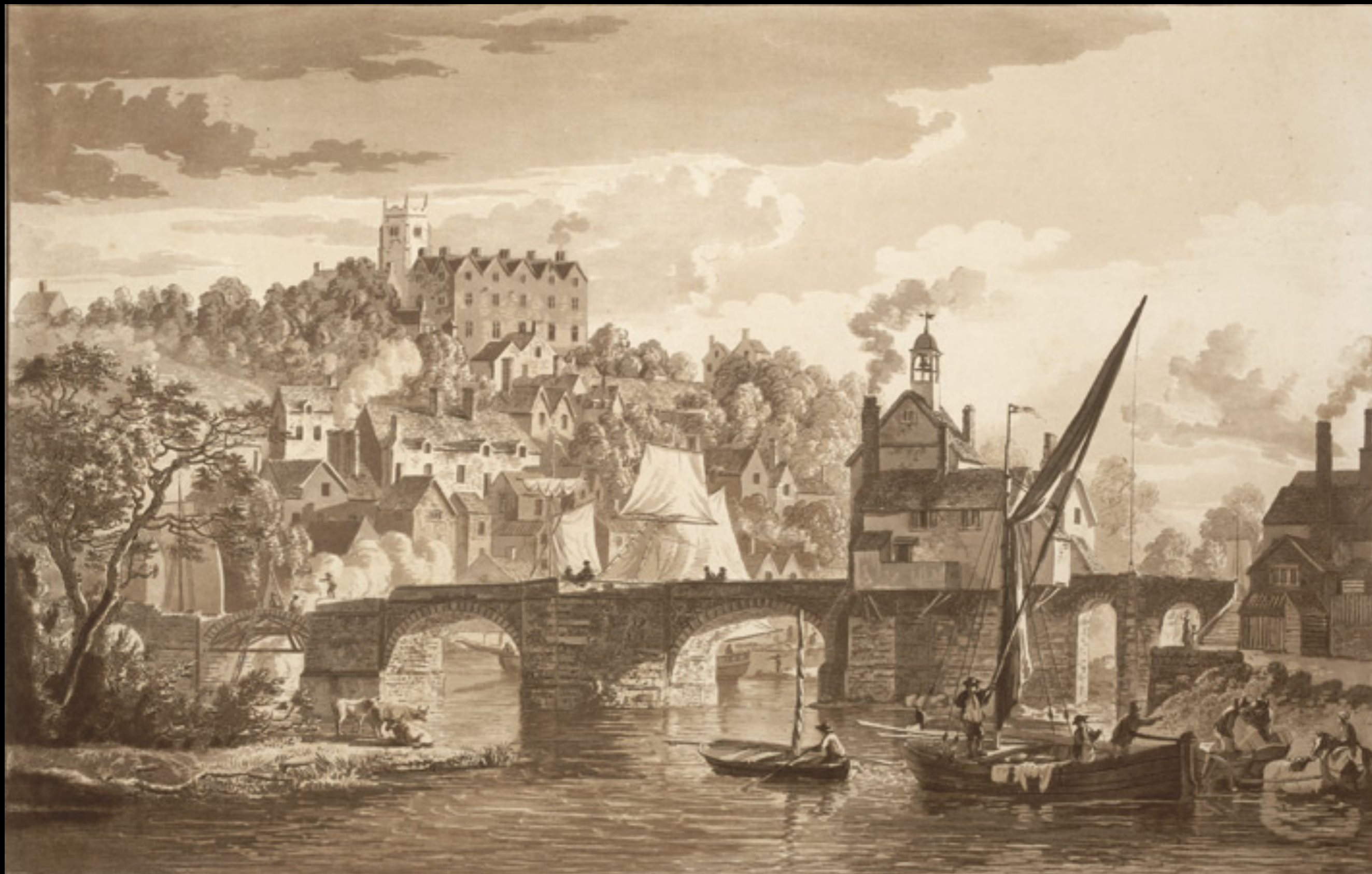
Bridge North Paul Sandby 1789 (The British Library)
