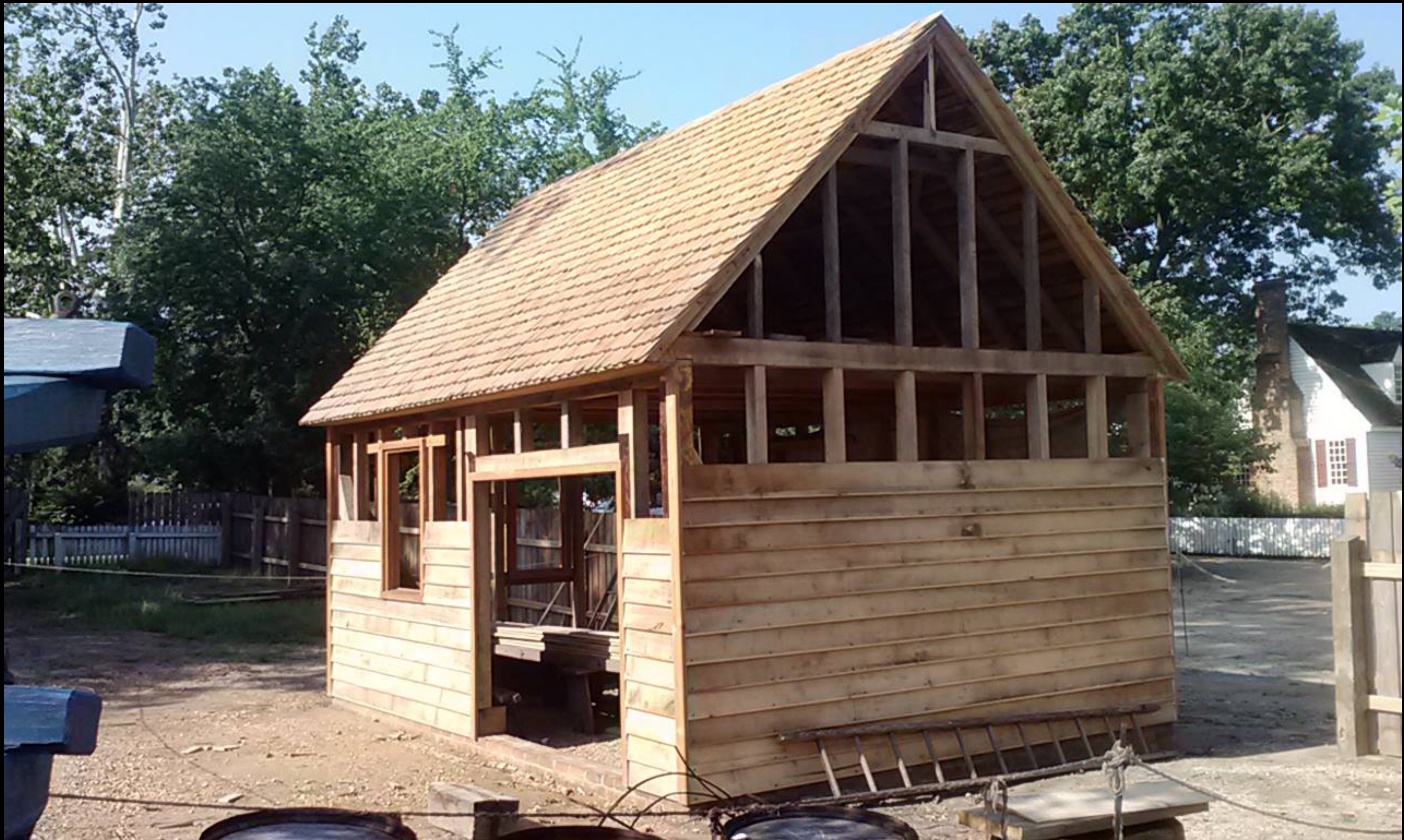
Recreated Timber Frame Construction Colonial Williamsburg
