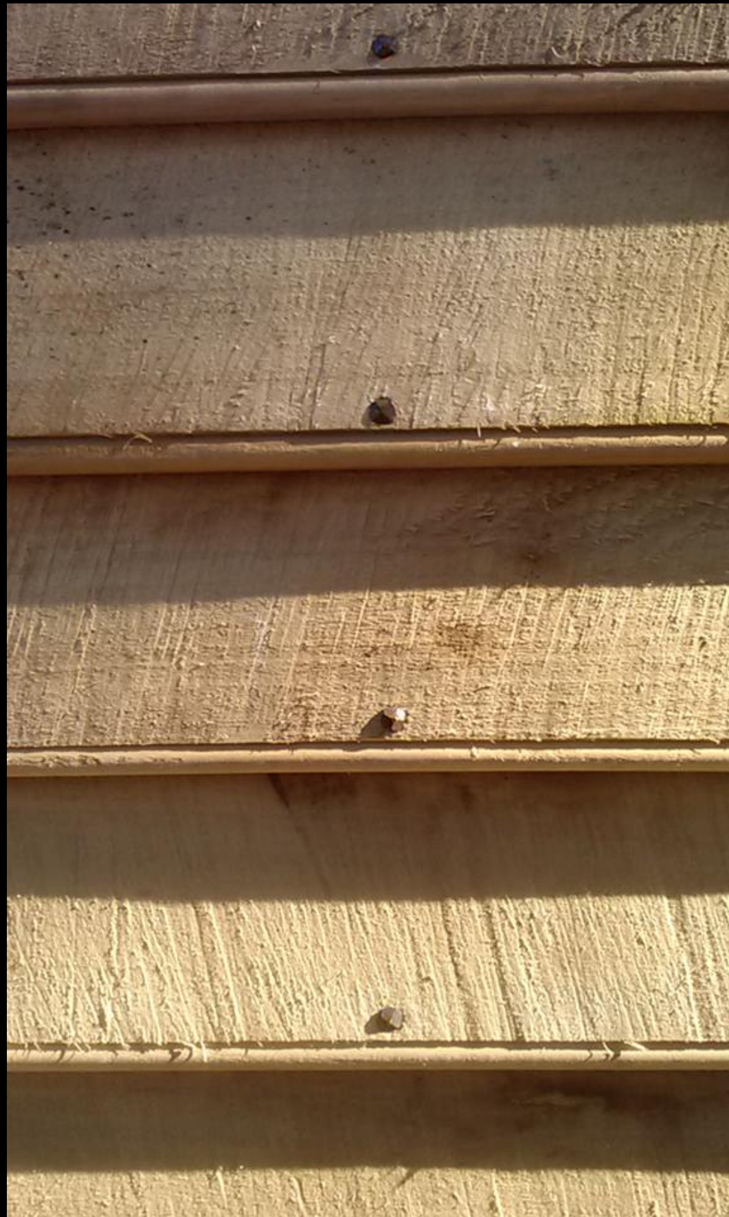
Recreated Timber Frame Construction Colonial Williamsburg
