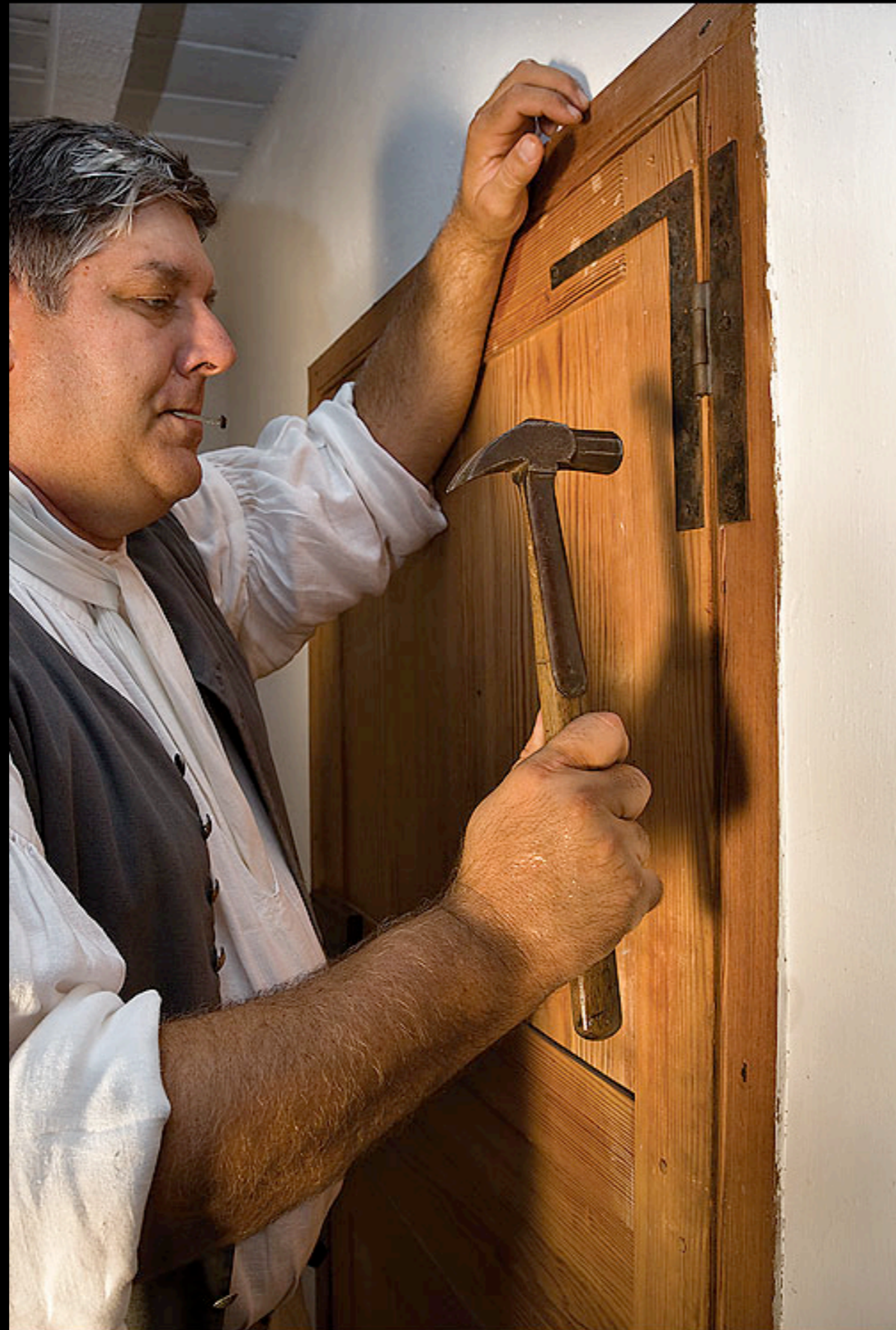
Recreated Carpenter applying a "HL" Hinge with a Claw Hammer (Colonial Williamsburg)
